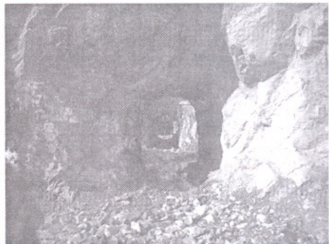
Fig.2 View of instrumentation tunnels driven across the ledges
