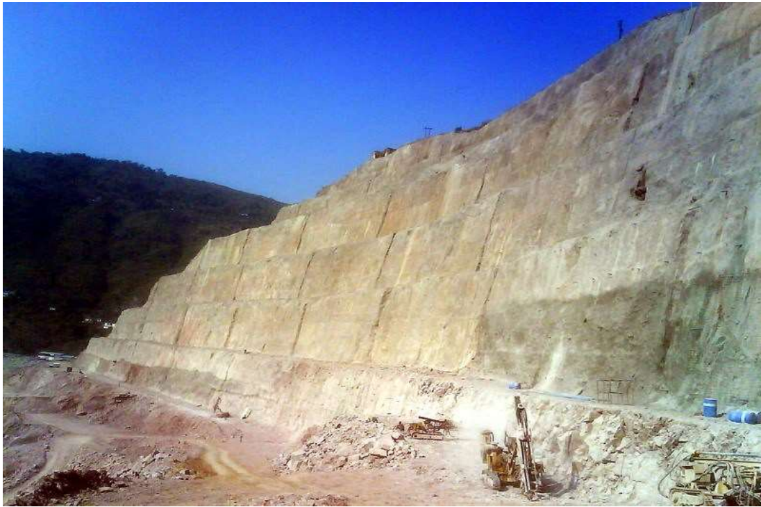
Fig.9: Benches formed by Pre-split Blasting at Kol Dam Project
