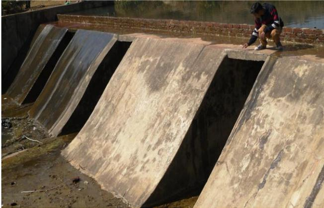
**Fig.6.2: Front view of the constructed check-dam**
