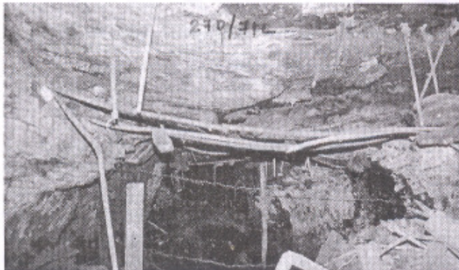
Fig.10: Roof instability during development of galleries at deeper cover
